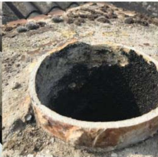
Rookgasafvoer stal 1
