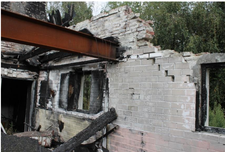
Later aangebrachte stalen liggers
