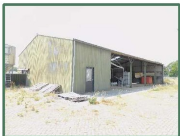
Te slopen loods
