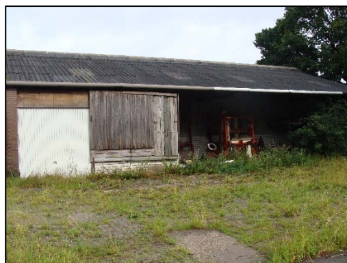
Foto 4. Te slopen loods
