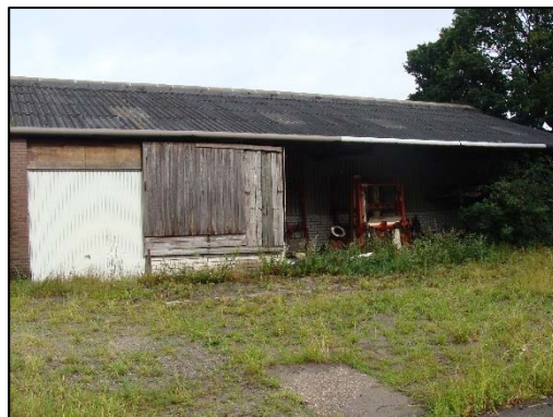
Foto 4. Te slopen loods
